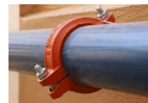
GROOVED COUPLER NEEDED WITH GROOVED PIPE
